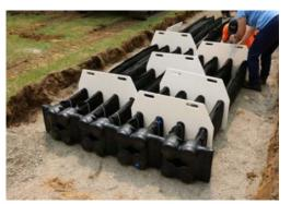
7. Once the fins are placed on the surface of the system sand and the distal end manifold system and/or end caps are connected to the fins per design, additional system sand shall be ladled between and to the top of each of the fin rows and lightly compacted by walking in the sand after placement for fin stabilization and support. Backfilling in a progressive
