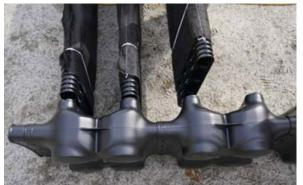
Next, working down the length of the bed begin connecting conduits end to end using the integrated snap lock joints to create rows to the specified bed length.
