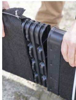
Fin rows shall be installed level to within +/- 1/2 inches (total 1 inch tolerance) of the specified elevation. A laser level or transit is recommended to ensure proper alignment.
