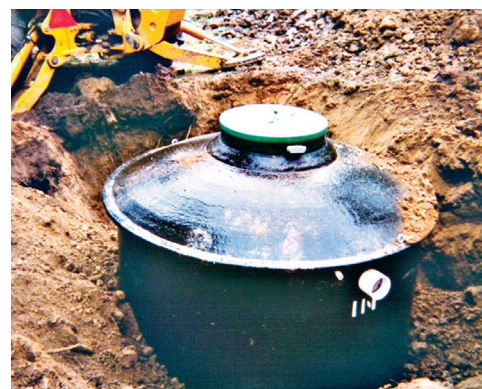
ECOPOD-C treatment tank installation
